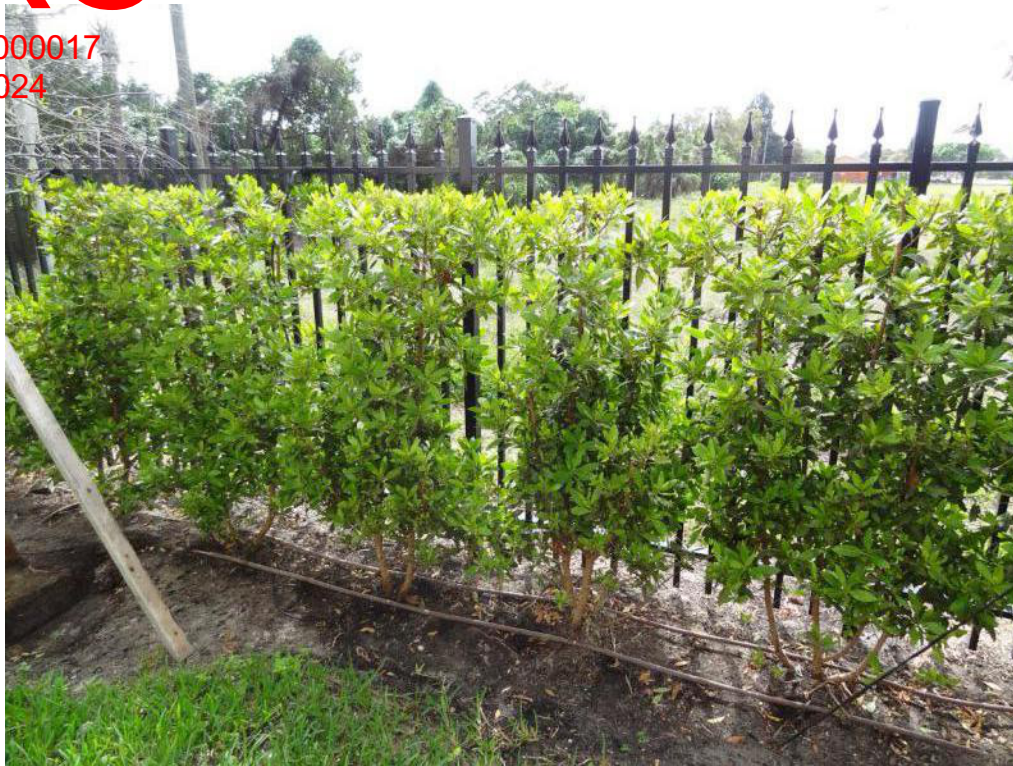
The fencing has a pointed topping to deter and dissuade climb overs.
