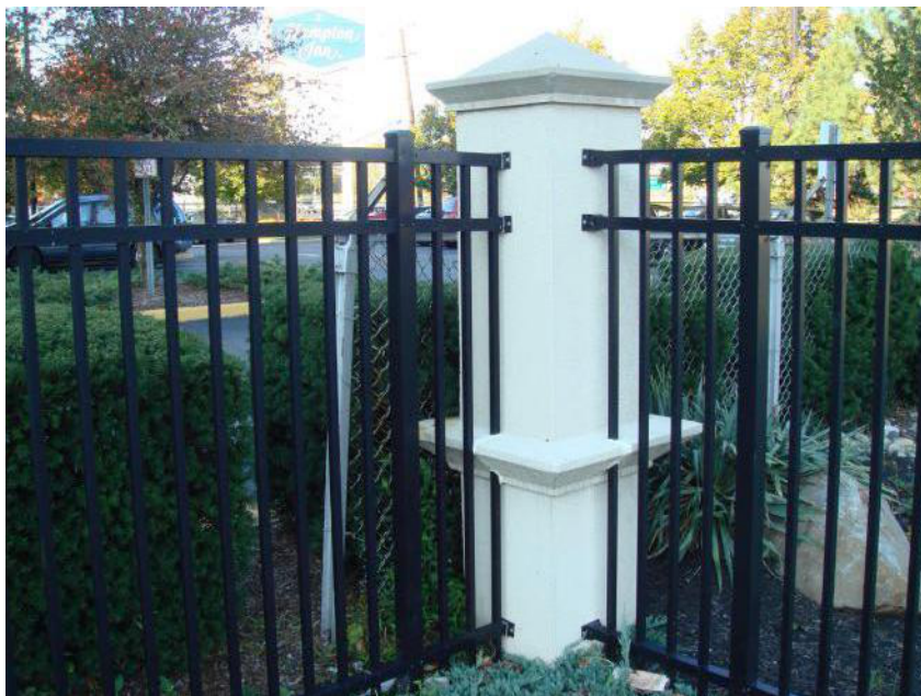
An example of very poor security fencing, because the post serves as an easy climbing ladder to get over the fence quickly,
